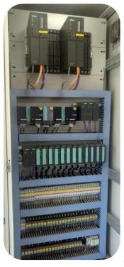
1). Main Control: liquid level control of boiler, water tank, and oil tank; steam pressure control; boiler system pressure control; temperature control, etc. Manual/automatic control of burners, pump valves, and other equipment, master, and backup switching. Water pump start and delay shutdown, water pump running status detection, and burner interlock.
