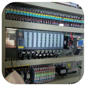
1).Main Control:liquid level control of boiler,water tank and oil tank;steam pressure control;boiler system pressure control;temperature control,etc.Manual/automatic control of burners, pump valves and other equipment,master and backup switching.Water pump start and delay shutdown, water pump running status detection and burner interlock.
